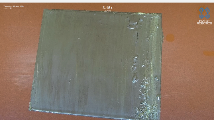
A new crack in a previously repaired patch. Residue that gets stuck in the cracks will eventually cause blisters beneath the repaired patch.
