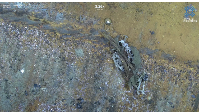
Contamination and corrosion in a CO2 vessel.
