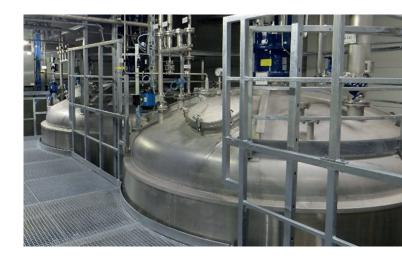
That is why these vessels have now for the third year running been inspected by Invert's remote camera system. Efficiently, thoroughly and avoiding all confined space access.
